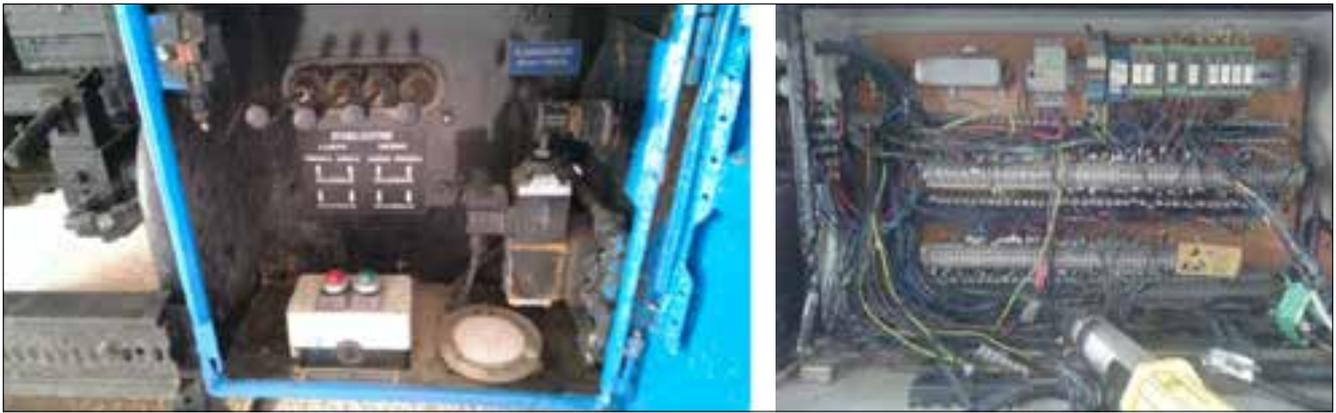
**Figure 2.** Cabinet for levelling process and main distribution cabinet before reconstruction
